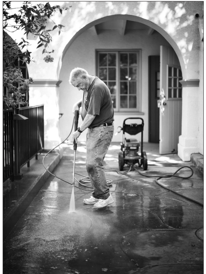
Bob Wright power washes the church walkways during one of two church workdays held this year.
